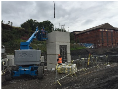
1 Lift Shaft No1 under construction
