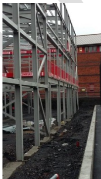
5 Steelwork adjacent to school building
