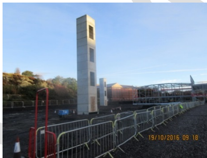
3 Lift shaft No.2 completed
