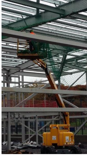
7 Erection of safety netting prior to completion of the roof works
