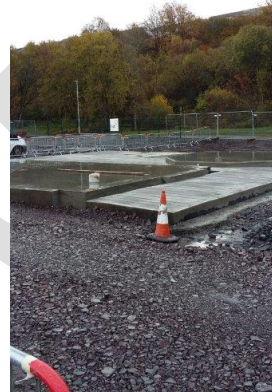
10 Concrete slabs for external buildings completed
