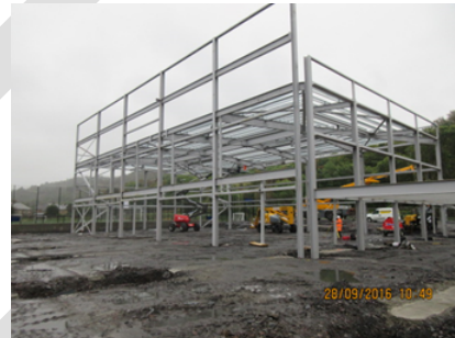
2 Games hall steelwork
