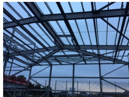
6 Sports Hall roof steelwork in place
