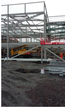
9 Commencement of steelwork for main building outwith sports hall
